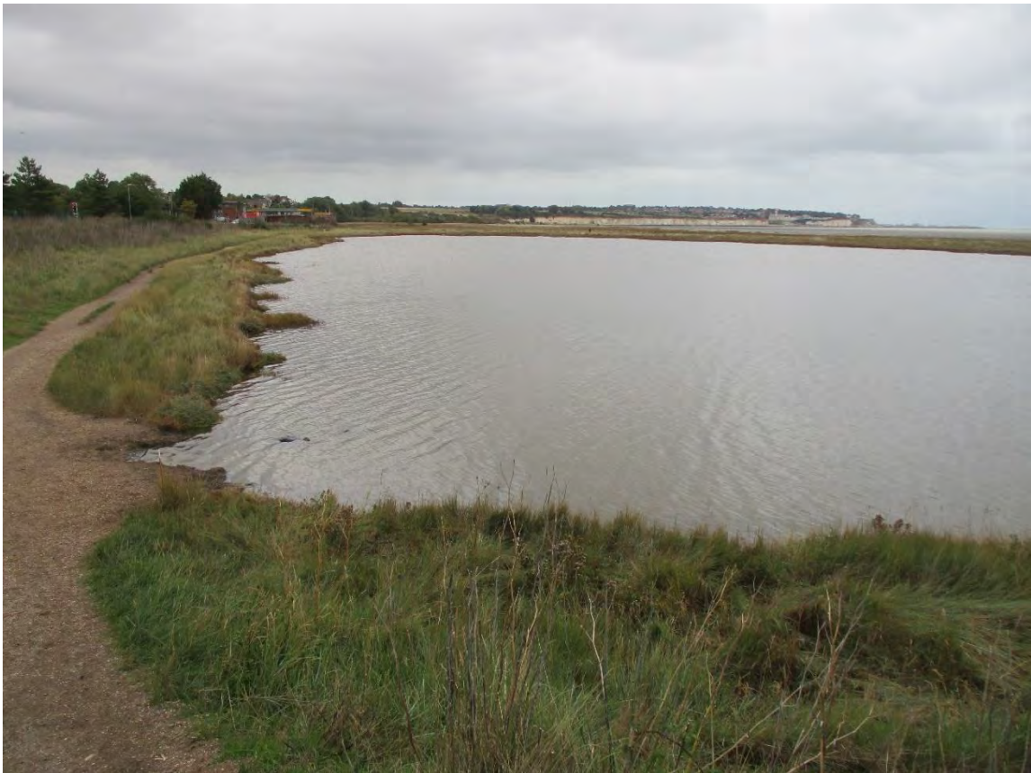
Photograph A3.32 The landward side of the lagoon, showing high water level
